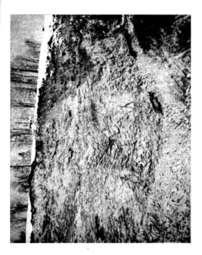
Figure 5. Zone of roof collapse above a deep mine. Former confining bed is now part of the aquifer (source bed B) which has a relatively high coefficient of permeability and contains a free water surface.
